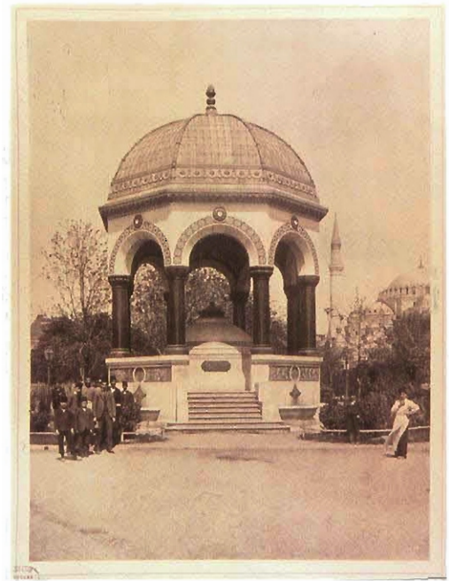
Fig. 9. Photograph of the Kaiser Wilhelm II Fountain at the Hippodrome, Istanbul. (After Gurlitt, Die Baukunst Konstantinopels , pl. 39a)
